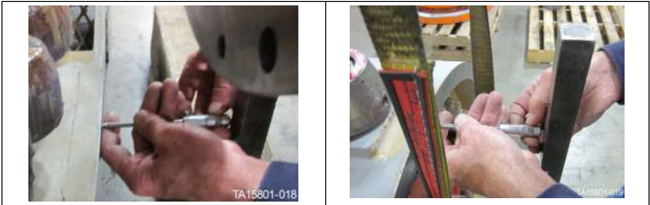
Figure 134. Measure "adapter to stator dimension" between face of rotor and face of generator pole ring
