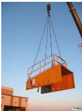
Figure 57. Hoisting the hood assembly
