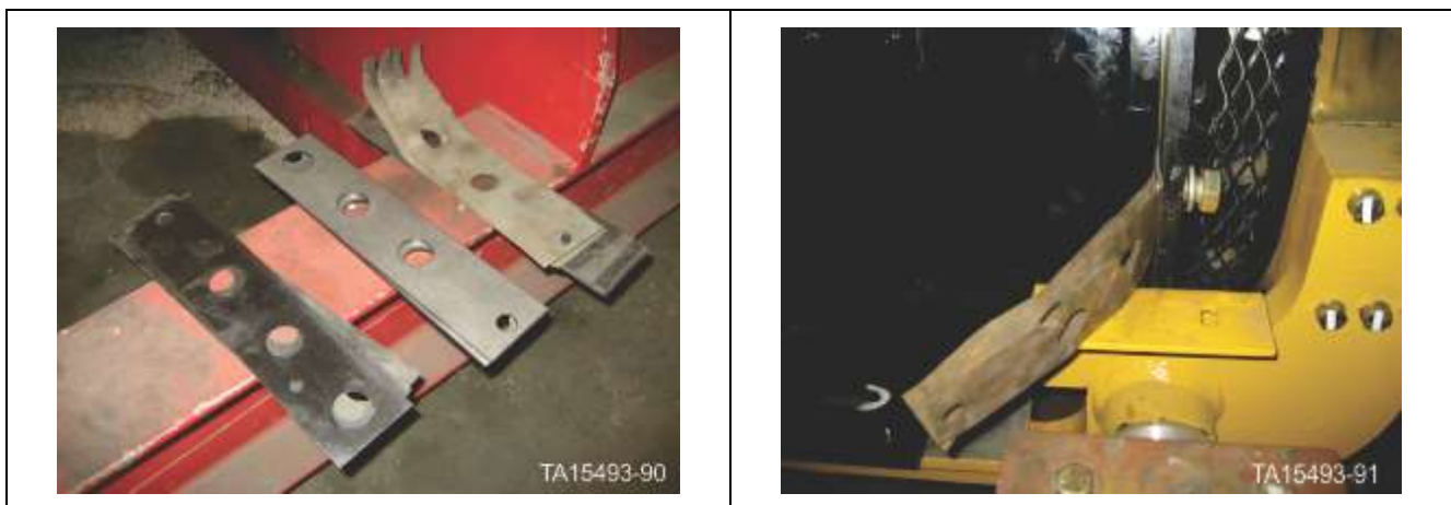
Figure 188. Install shims on both sides
