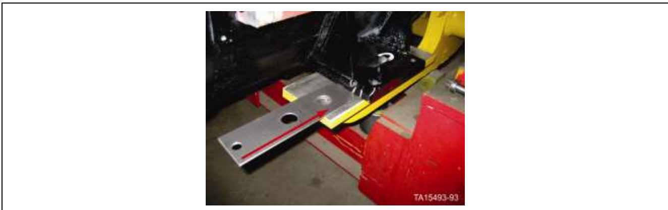
Figure 190. Installation of the shim pack at the generator mount foot
