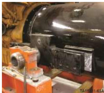
Figure 293. Join motor and generator together
