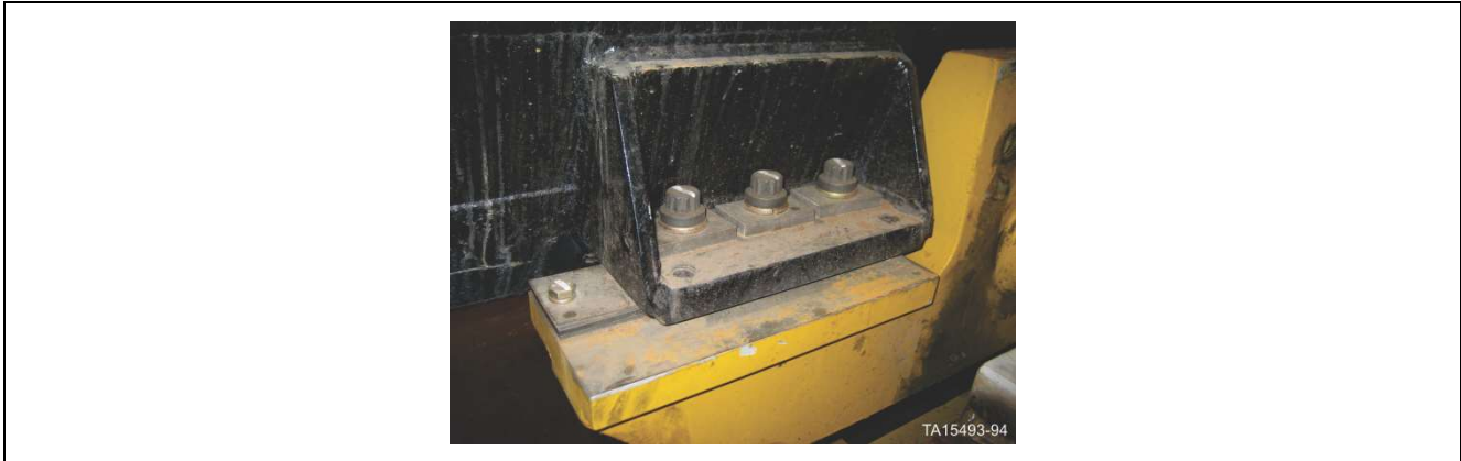
Figure 191. Shim pack installed at the generator mount foot
