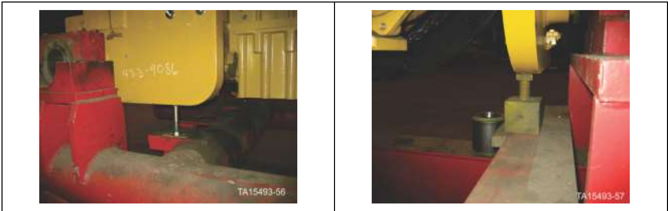
Figure 86. Support jacks under rear engine mount
