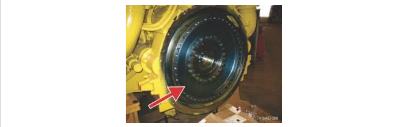
Figure 159. Measurement of radial runout of engine flywheel - Tier 2 DD/MTU
