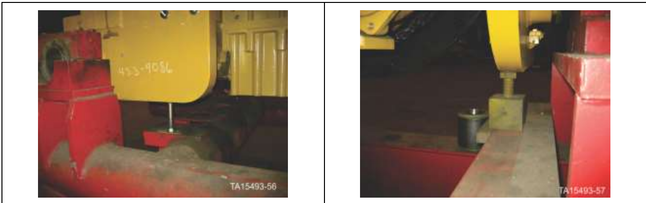
Figure 148. Jack bolt placed directly under the engine mount
